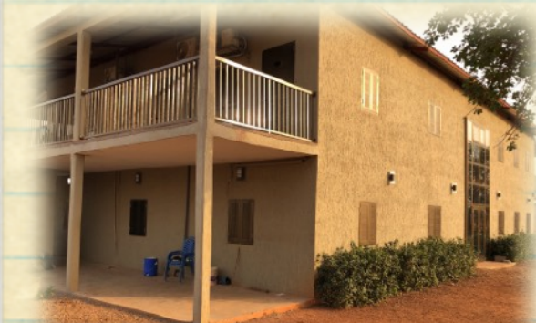
Hope Radio phase 2 Construction of 2nd story 95% complete
